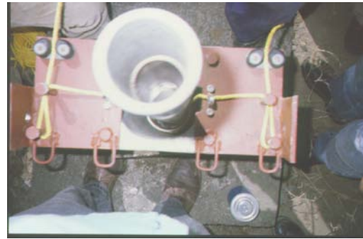
Figure 2. Rope Guide Plates for Installation, Viewed from above riser pipe column
