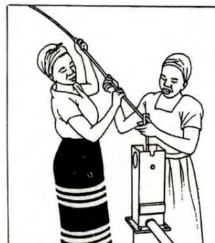
24. Put the plunger and pump rods back together and lower them down the borehole.
