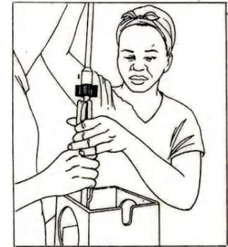
12. Slide the rubber centraliser where the rods join.
